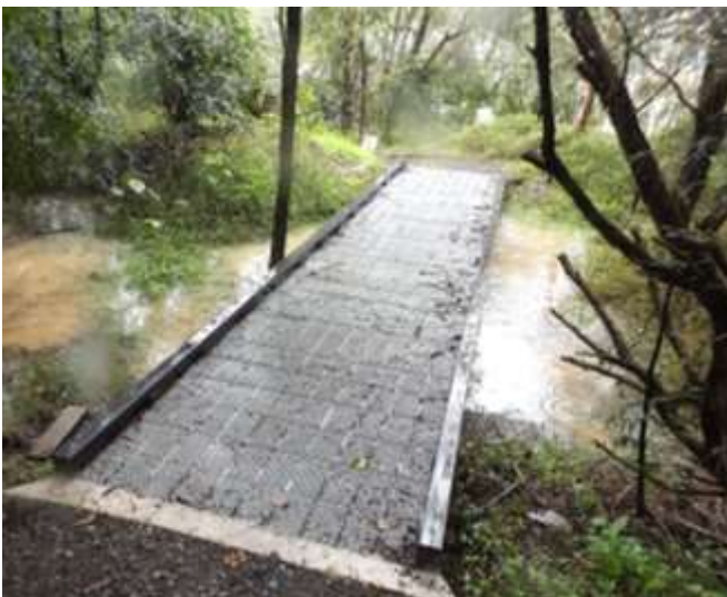
New Walkway in Room 5 after recent heavy rain
