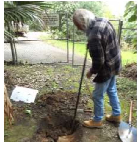
Grahame at work on repairing break in drain pipe near Useful Plants Garden
