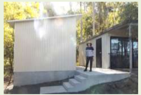
Hazel proudly showing off the new amenities block building
